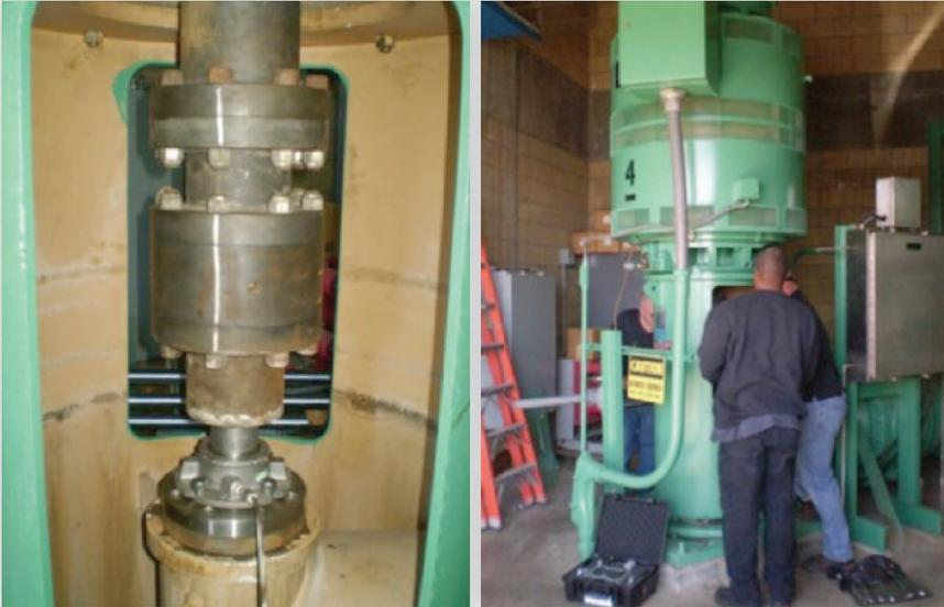
Since we didn’t want the coupling and shaft stiffness to influence the alignment readings, the decision was made to remove the coupling bolts and rest the impeller in the pump bowl, treating the pump as a non-rotating shaft. The other option was to loosen the coupling bolts
