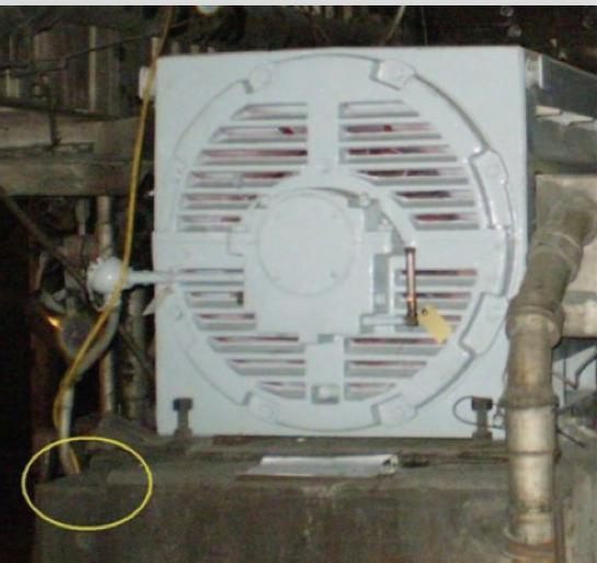
Initial inspection of the motor installation revealed a slight bit of concrete to have been broken off from the left rear and right front corners of the foundation under the outer edges of the motor base. There were no shims under the motor feet. The gear coupling was already assembled so 0.050" thick shims were placed under all motor feet as a starting point.
