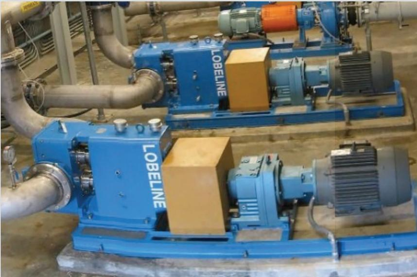
We were asked to bring turn down bolts and perform the final alignment. We packed up our Fixturlaser GO Pro and undercut bolts then headed out for some in-the-trenches training.
