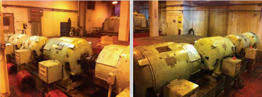
This assessment is tackled by measuring the alignment condition from the induction motor to the first piece north. After this is measured, then the remaining pieces going north will be measured by using the Machine Train program. With the Fixturlaser XA Pro, we can make the machine template with machine names
