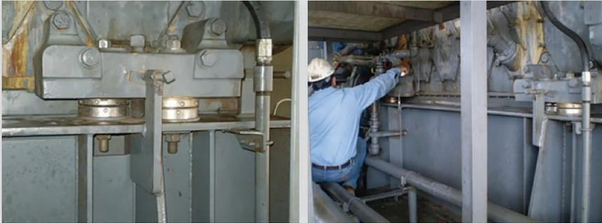
The Verti-Zontal process is modified slightly by taking the three alignment measurements from top to bottom (12 o'clock, 3 o'clock and 6 o'clock, for example) vs. side to side (9 o'clock, 12 o'clock and 3 o'clock) as when aligning a “shimmed” machine. After the results are analyzed press the shim icon as you normally would and note the feet position. This is the vertical position of the movable machine at the feet **BEFORE** the hold down bolts are loosened. Then press the live adjustment icon.
