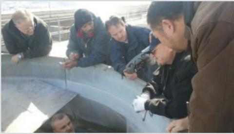
This was a Marley cooling tower, with a 60 HP motor, connected to the gearbox by a 48" spacer shaft.
