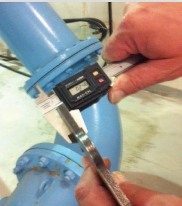
We also checked each shim in several locations to make sure the thickness was uniform. If the shim had more than a 2 mil variation, we would discard it. The reason is we have a 2 mil soft foot tolerance and would not want to create an angular soft foot because of shim quality. We also would recommend that you mic all shims 50 mils and thicker. The thicker the shim, the more likely there are variations. We have seen 125 mil shims as thin as 114 mils, 11 mils thinner.
