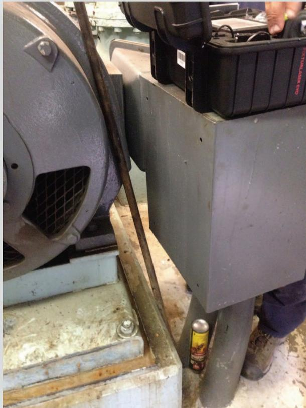
The junction box is against the breaker panel. On this one we were able to pull the breaker panel far enough away to align the equipment. It still needs to be modified
