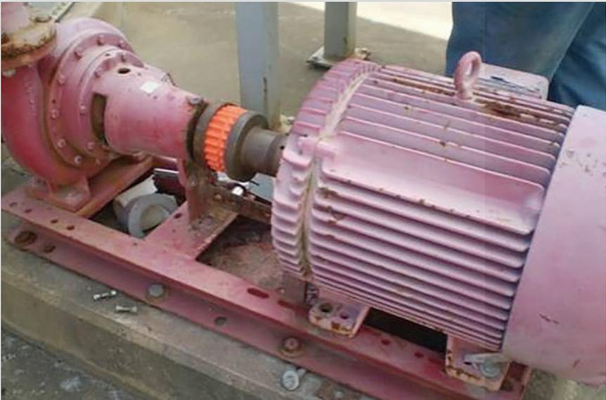
As the hold down bolts were tightened (in a cross torque pattern) the horizontal offset would change to approximately 5 mils at 50% torque then 8 mils at 100%. After 2 attempts the same amount of horizontal movement took place. The students were bewildered. The machine had no soft foot, the coupling backlash had been neutralized and there was no other looseness.
