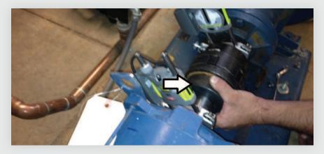
Then rotate the sensor to 3 o'clock to take the third measurement. When the sensors pass 12 o'clock, switch the engagement to the pump (driven) side. This will keep the coupling engaged in the same direction throughout the measurement process.
