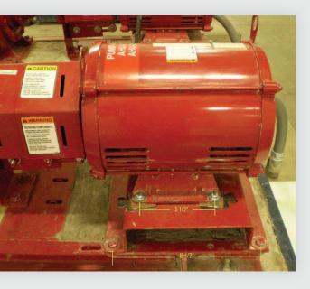
So for this motor alignment we adjusted the Verti-Zontal Compound Move slightly.
