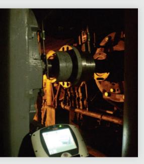
Initial inspection of the motor installation revealed a slight bit of concrete to have been broken off from the left rear and right front corners of the foundation under the outer edges of the motor base. There were no shims under the motor feet. The gear coupling was already assembled so 0.050" thick shims were placed under all motor feet as a starting point.
