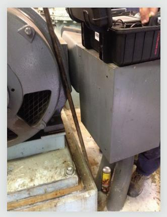
The junction box is against the breaker panel. On this one we were able to pull the breaker panel far enough away to align the equipment. It still needs to be modified
