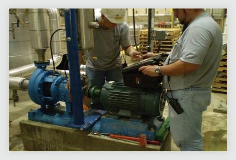
During a recent GO Pro training class, an alignment check was performed on a Goulds 3196 pump, driven by a 20 HP electric motor at 1765 RPM. The pump runs intermittently– only several hours a day.
