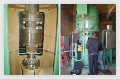
Since we didn't want the coupling and shaft stiffness to influence the alignment readings, the decision was made to remove the coupling bolts and rest the impeller in the pump bowl, treating the pump as a non-rotating shaft. The other option was to loosen the coupling bolts just enough for an approximate 0.050" gap between the coupling hubs, which would still allow pump shaft rotation but would have eliminated the coupling stiffness issue.
